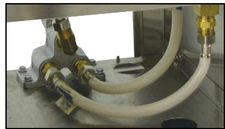
Heater feeds hot and cold water supply to the Valve in Pedestal Base and Knee Valve Units (Pedal Valve Shown)
