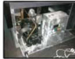
PULL OUT CONDENSING UNIT ON SELF CONTAINED
